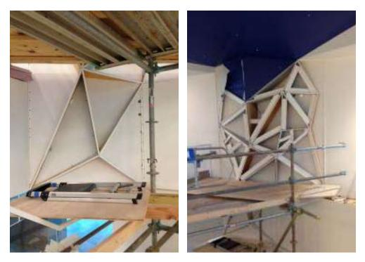
In this project, the profiles cover the upper part of the main staircase and the ceiling of the top floor. They were fixed to a wood and metal substructure based on a CLIPSO workshop drawing and then manufactured on site by the US approved installer: Fabric Wall Concepts.
