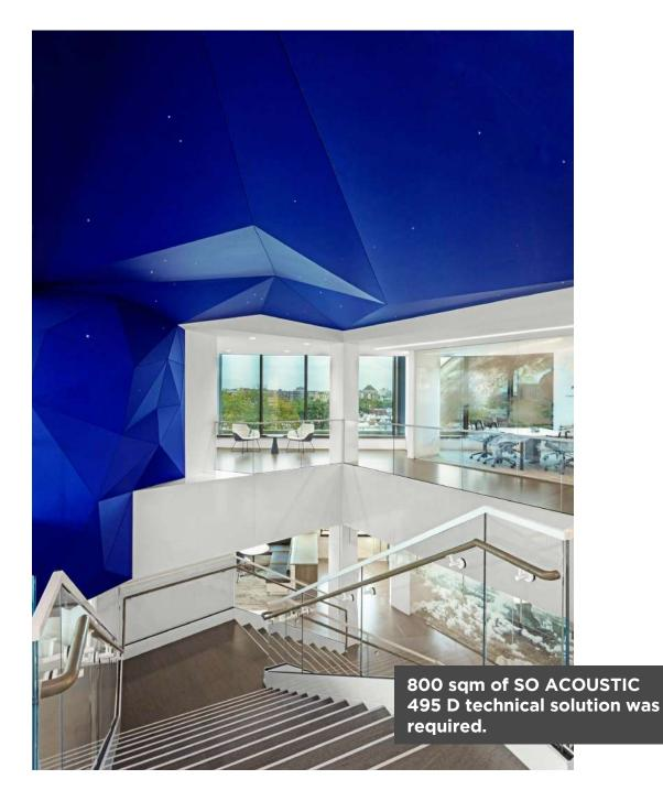
The structural framework had to be rigid enough not to deform throughout the rather complex installation process of all the adjacent surfaces. The biggest challenge was to achieve a clean fabric edge when up to six pieces of profile (10mm thick white P-CC) intersect at a single point on several different levels.
