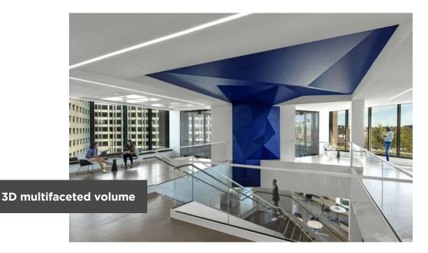
The versatility of the CLIPSO system, the SO ACOUSTIC & SO AERO coverings ranges and the know-how of all the people involved made it possible to achieve the architect's main objective: to create a multifaceted 3D volume in a specific deep blue color, dotted with fiber-optic lighting. The result is a unique space that looks like a vast starry vault, a symbol of the AGU's geophysical mission.
