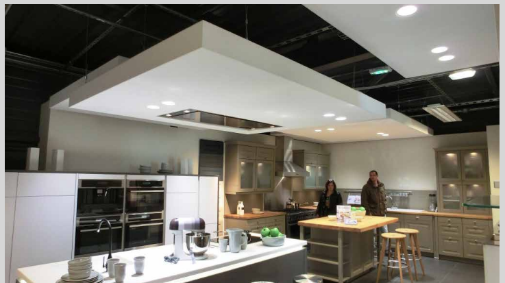
Sales area - FRANCE XXL acoustic frame with light integration and hood Installation: KALLISTE
