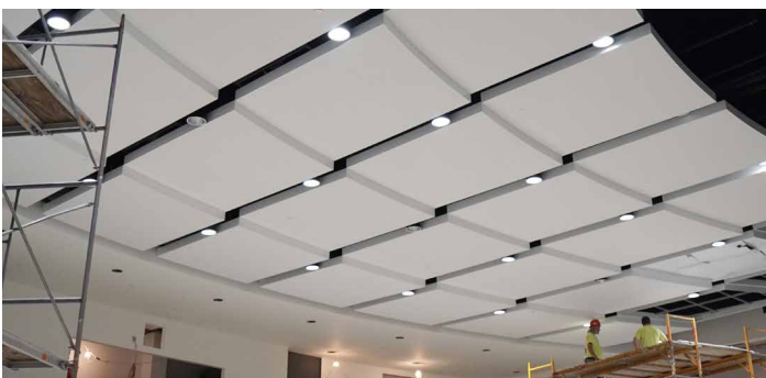
Ariel Corporation Auditorium - USA Custom acoustic frames, colour 'pepper' Installation: Ketchum & Walton Co.
