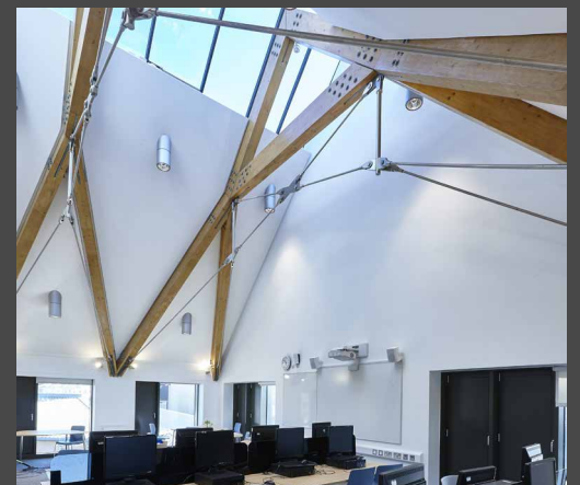
Library - THE UNITED KINGDOM Acoustic ceiling between beams Installation : Acoustic GRC
