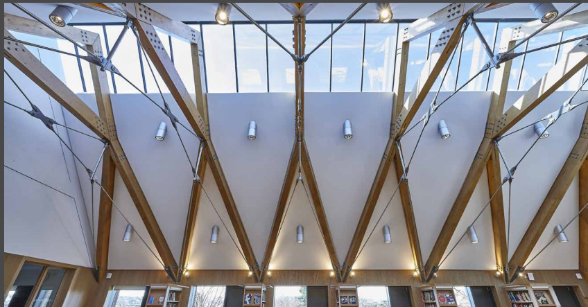
Library - THE UNITED KINGDOM Acoustic ceiling between beams Installation : Acoustic GRC
