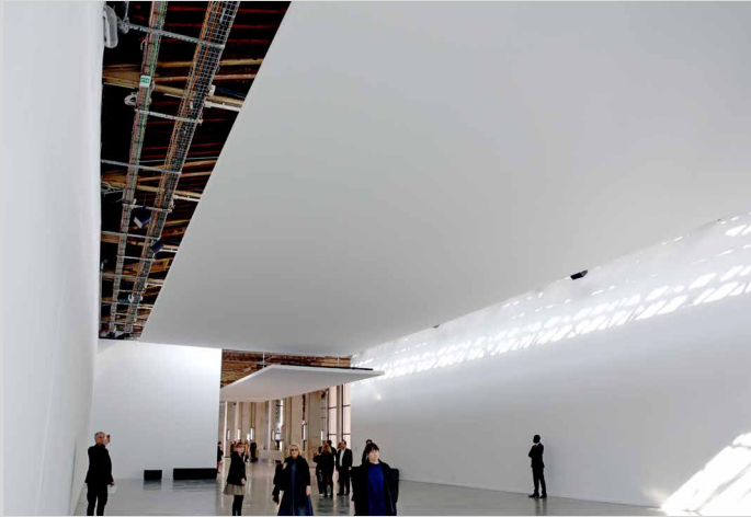
Anywhere, Anywhere Out of The World exhibition at the Palais de Tokyo - Paris - FRANCE - Suspended acoustic ceilings Artist: Philippe Parreno - Installation : CLIPSO
