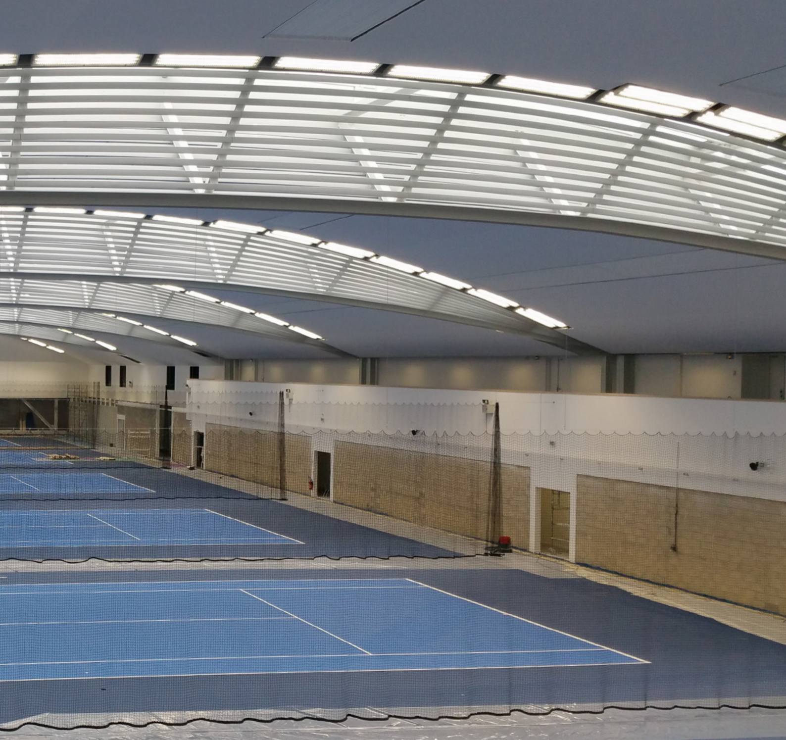
Training centre of the French Tennis Federation - Roland Garros - FRANCE - Architect: Marc Mimram
